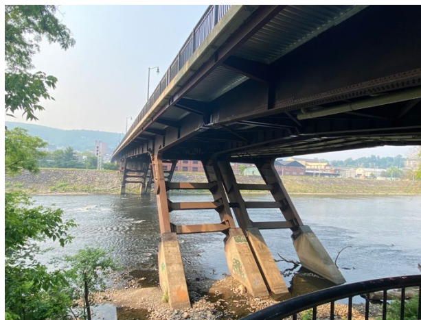
Figure 7: Fahy Bridge center span over the Lehigh River.
