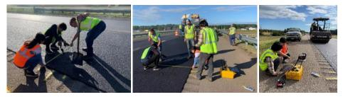
Figure 8 SmartRock installation and data collection in Indiana project
