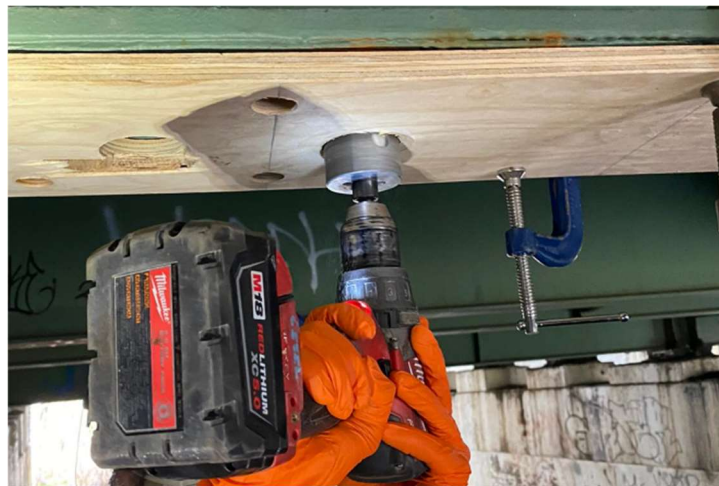
Figure 69. Diamond-coated core saw used to drill the CFRP composite system.
