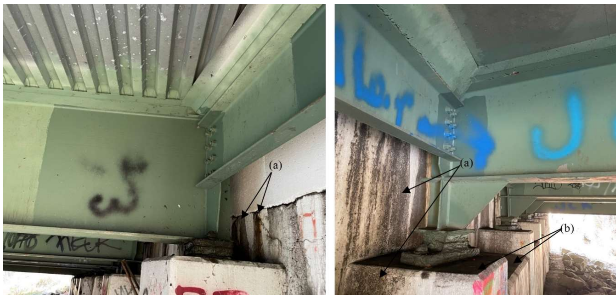
Figure 76. Damage to CFRP laminate from grit blasting.
