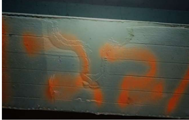
Figure 76. Damage to CFRP laminate from grit blasting.
