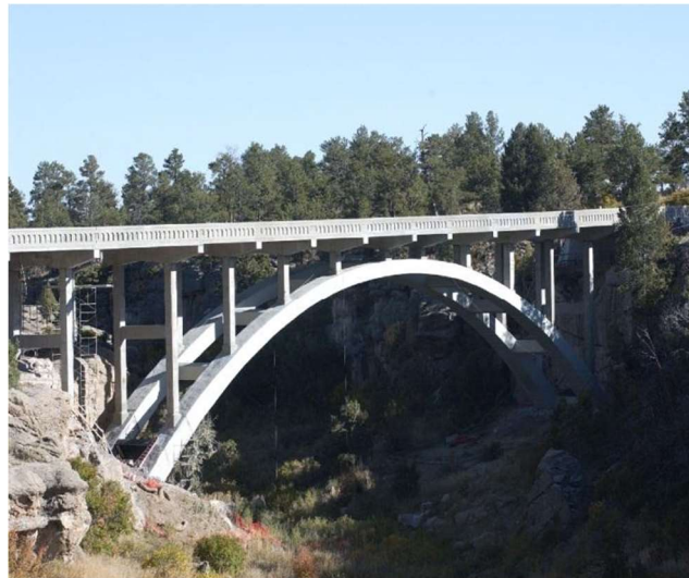
Figure 9. Castlewood Canyon Bridge after the 2003 repair where the pull-off tests were conducted.
