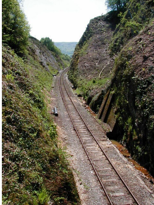
Figure 1.1. Example of a through-cut.
