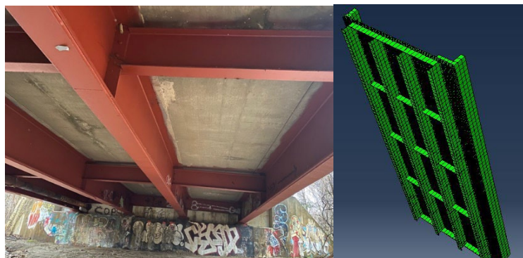
Figure 5: Underside of bridge superstructure photo (left) and ABAQUS model (right) of DE 1-213
