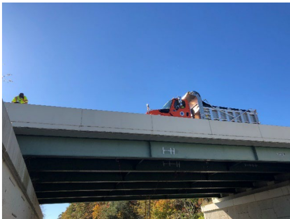
Figure 3: Loaded truck crossing bridge during a load test
