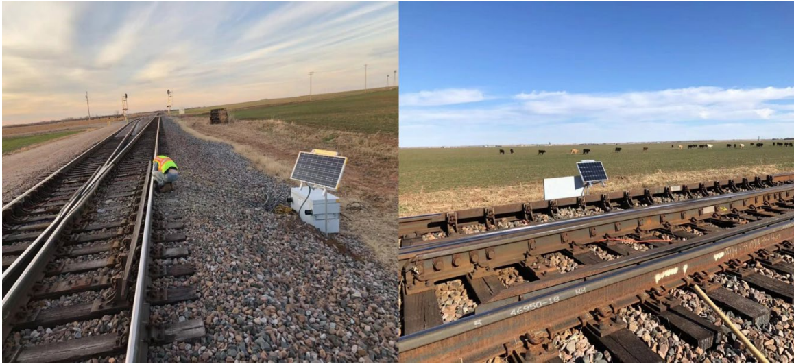
Figure 5. Photo showing the track layout where the SmartRocks were installed.
