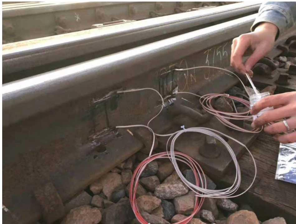
Figure 12. Four strain gauge channels attached to the field side of the rail.
