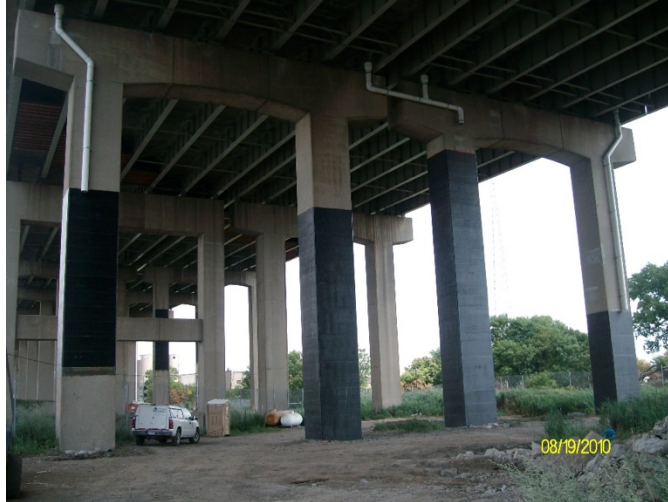
Figure 2. CFRP strengthening of bridge piers (Florida International University, 2019).
