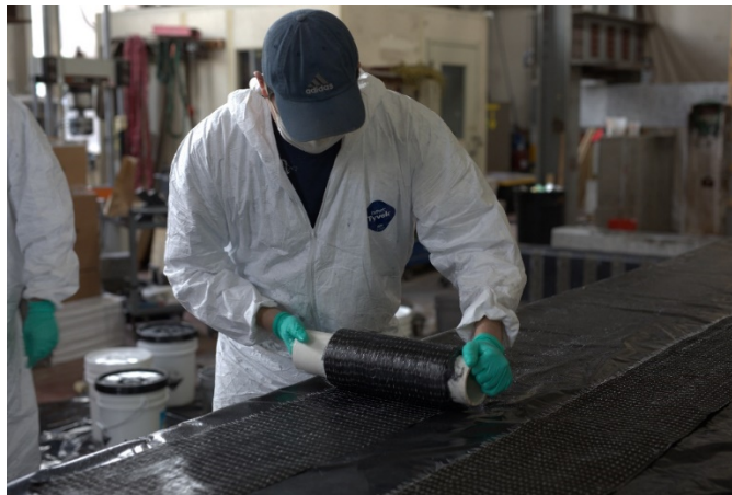
Figure 30. Rolling the saturated fiber onto a section of PVC.
