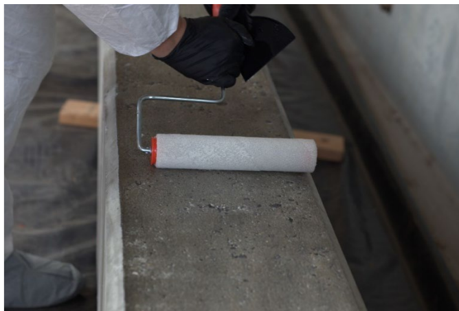
Figure 26. Applying epoxy to the concrete substrate using an epoxy roller.
