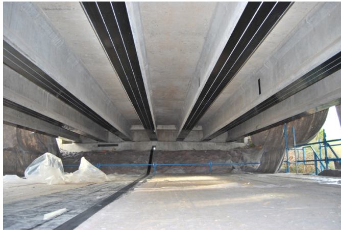
Figure 3. Flexural strengthening of bridge girders using CFRP (Concrete Protection & Repair Services, 2019).
