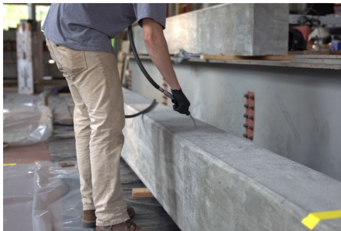
Figure 23. Cleaning the surface of the concrete with compressed air.
