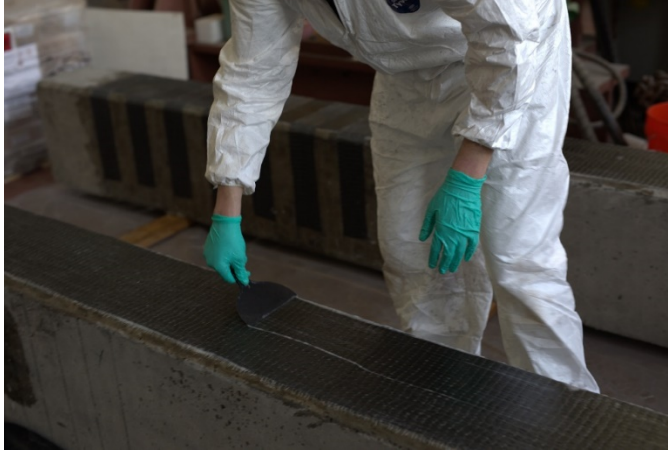
Figure 32. Smoothing the CFRP onto the surface of the beam using a putty knife.
