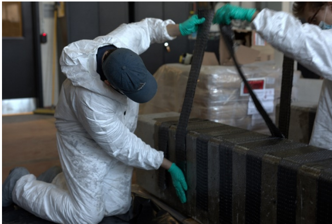
Figure 33. Installing U-Wraps onto the girder.
