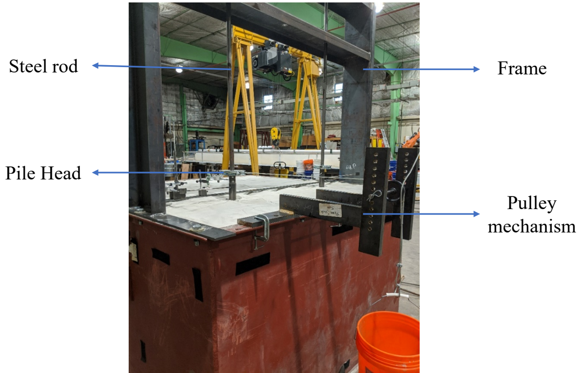
Figure 3.20. Pile after installation.
